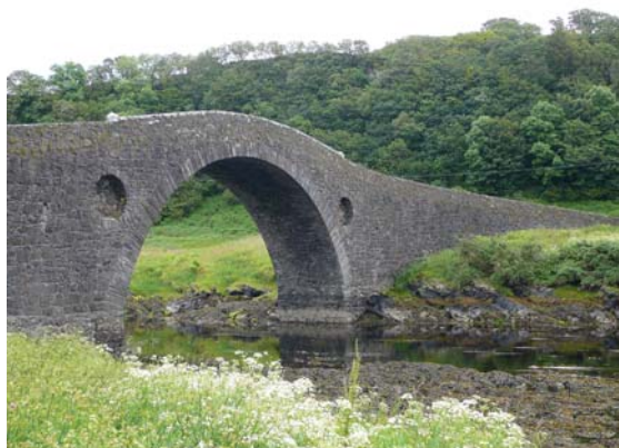
Clachen Bridge at low water – 10.5m
